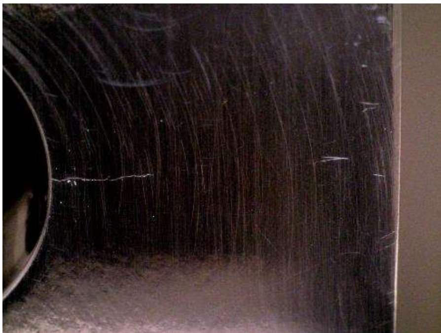
Figure E.12: Specimen CX140ED-2 under zero applied stress. Crack is approximately 0.140 inches in length and appears to be closed.
