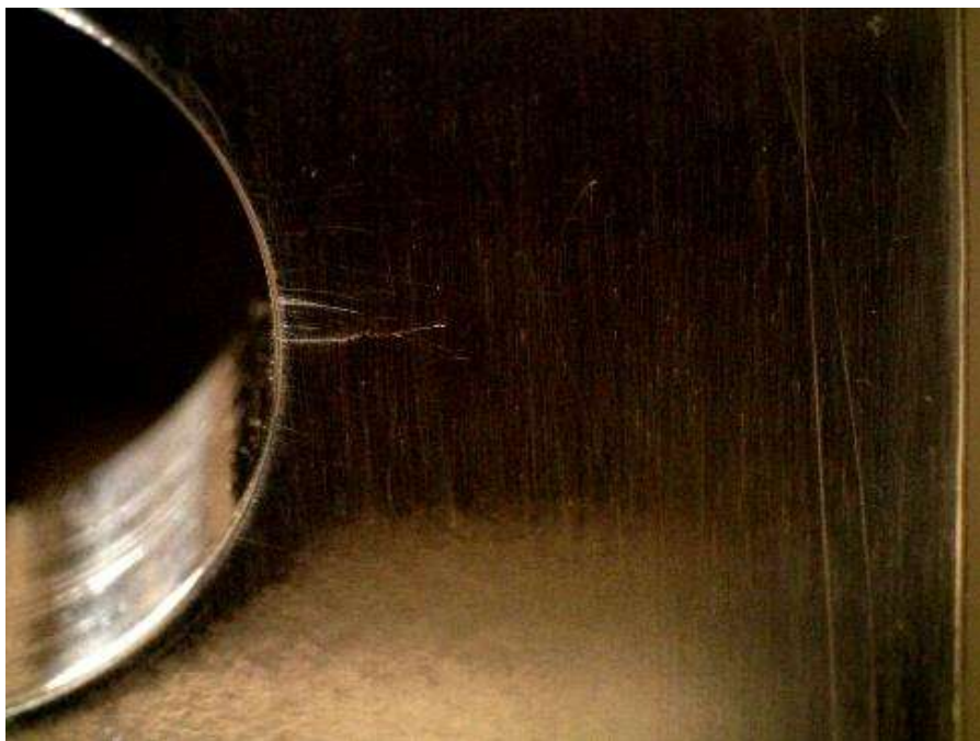
Figure E.2: Specimen CX130ED-2 under 3.3 ksi applied stress. Crack is approximately 0.103 inches in length and appears to be closed.
